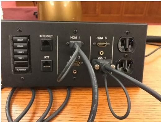
*There are input boxes at each attorney table as well as at the podium. These input panels can be used to integrate your laptop into the courtroom technology so you can display your laptop output on courtroom monitors.*
